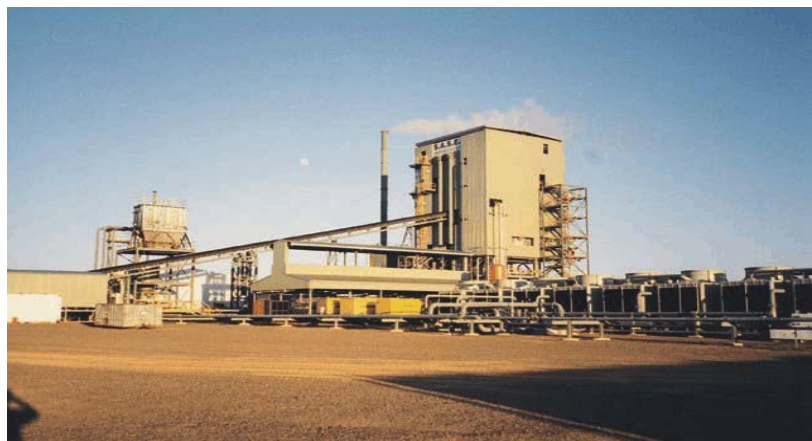
Cover Photo—Tapping the AusIron® Furnace
